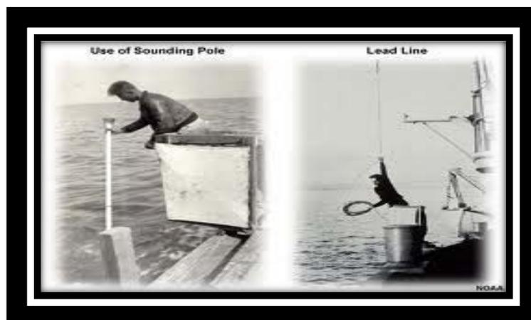
Fig 1-1 (Lead line and sounding pole method)
